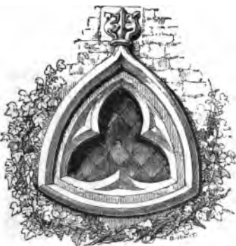
129. Cranford St. Andrew, Northants, c. 1320. Clerestory window of the form called a spherical triangle.
